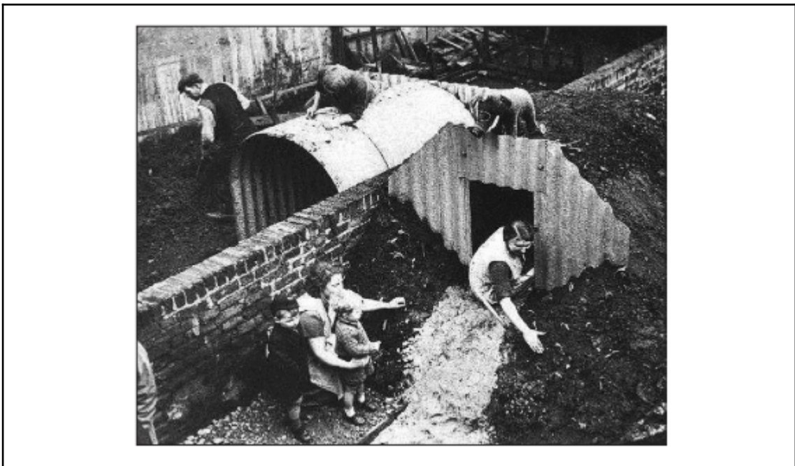
[A photograph of an Anderson Shelter supplied by the British government from May 1939 onwards.]
